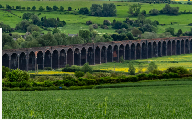
WELLAND VALLEY VIADUCT, RUTLAND
